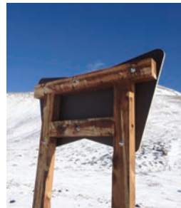
Wood Cross Braces
